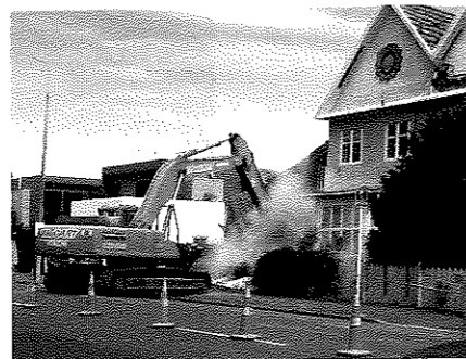
Recovery begins with the demolition of unsafe buildings.
