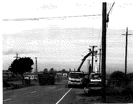
Build back better aims to reduce infrastructure vulnerability.
